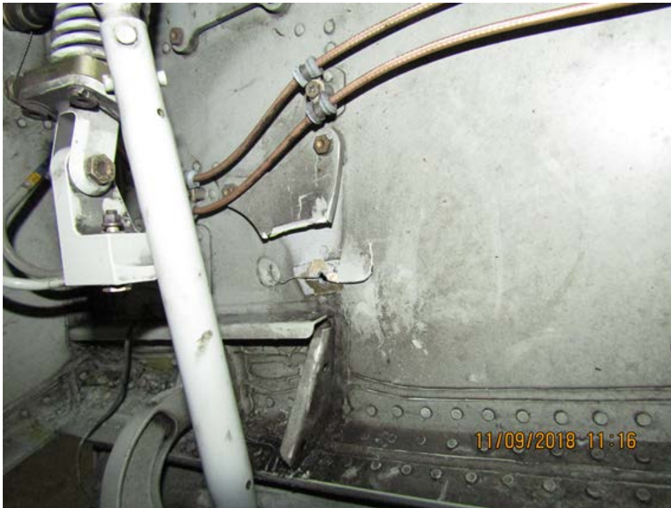
Figure 3: Broken bracket viewed from front showing bulkhead damage
