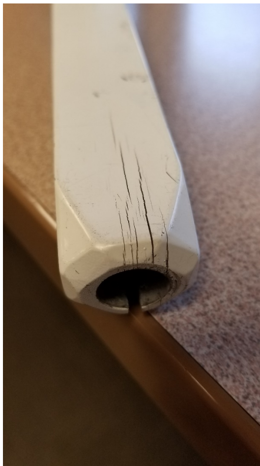
Fig 1: Lever cracking on both sides
